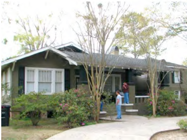
Oxford House - Cole 3565 Cole Drive Baton Rouge, LA 70806 8 Men • Established October 1, 2009
